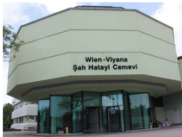
Alevi prayer house (Cem House) in Vienna, Schererstr. 4, 1210 Vienna: Sah Hatayi Cemevi, named after the Alevi mystic Sah Hatayi, whose praises of the 12 imams and cem rituals are still used by Alevi today. © Alevi Community in Austria (ALEVI)
